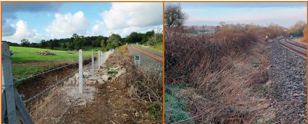
The photo shows the method of coppicing of Hedgerow along a section of track completed in 2014 (Limerick to Waterford Line).
