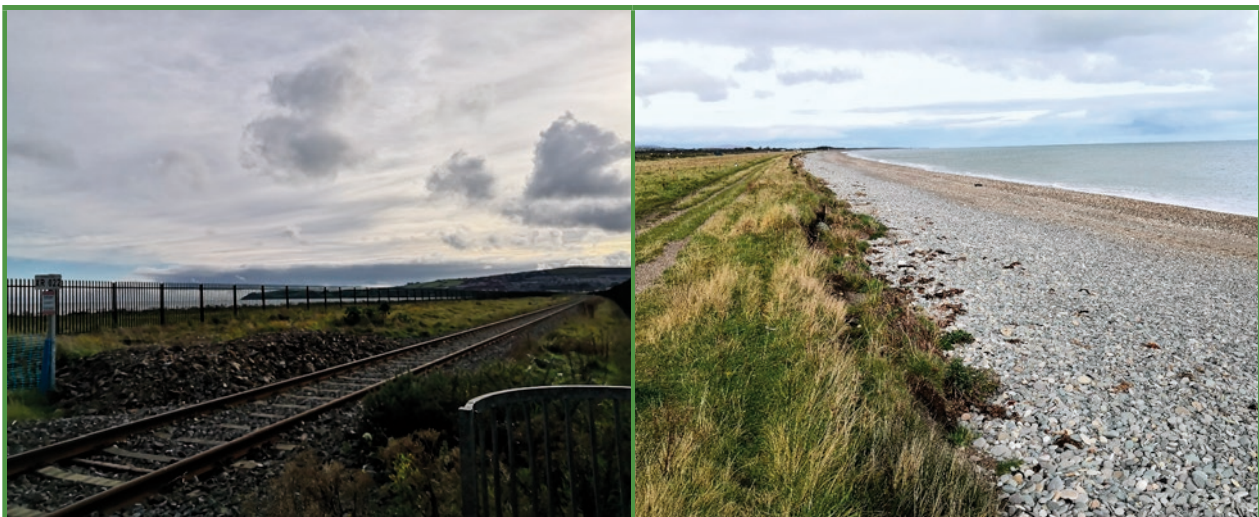
The active track above is the Shanganagh Junction to Wexford Line along the East Coast and in certain parts of track there is roughly 130m between track and the Sea.
