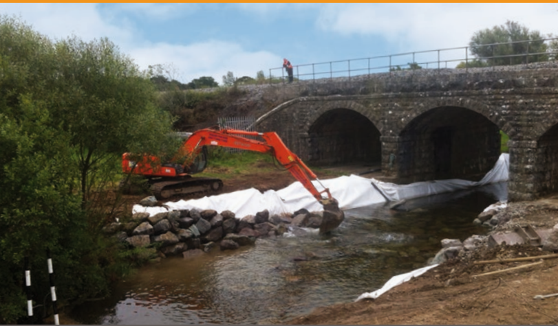
Case Study 2 – Scour remediation works in progress on the Dublin/Cork Line
