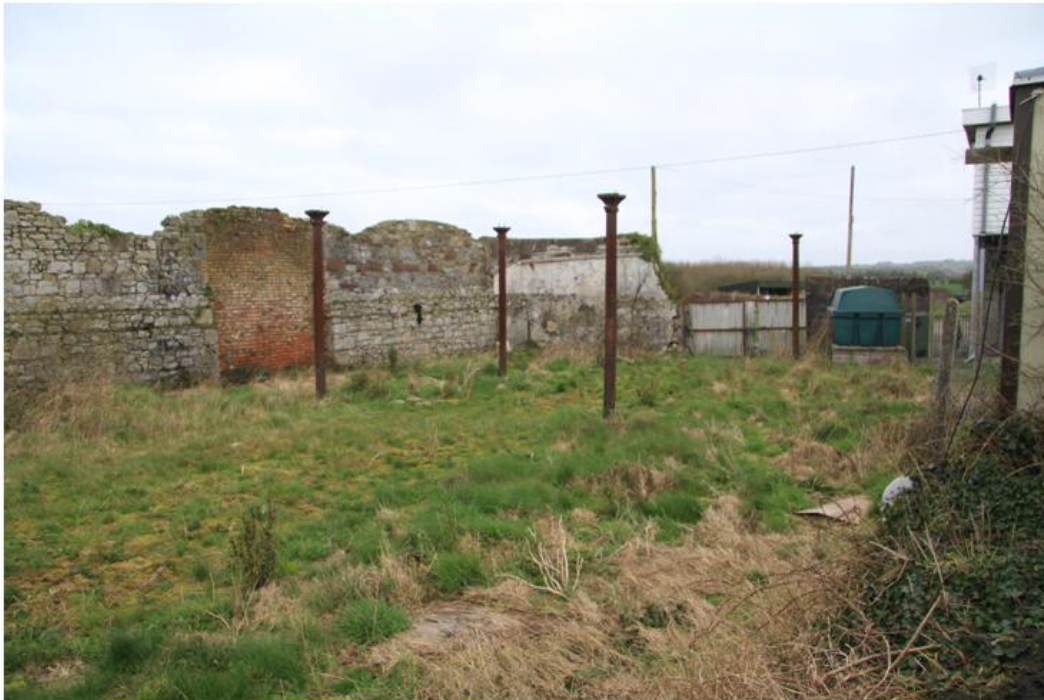
Plate 13: Western goods shed, seen from the south-east
