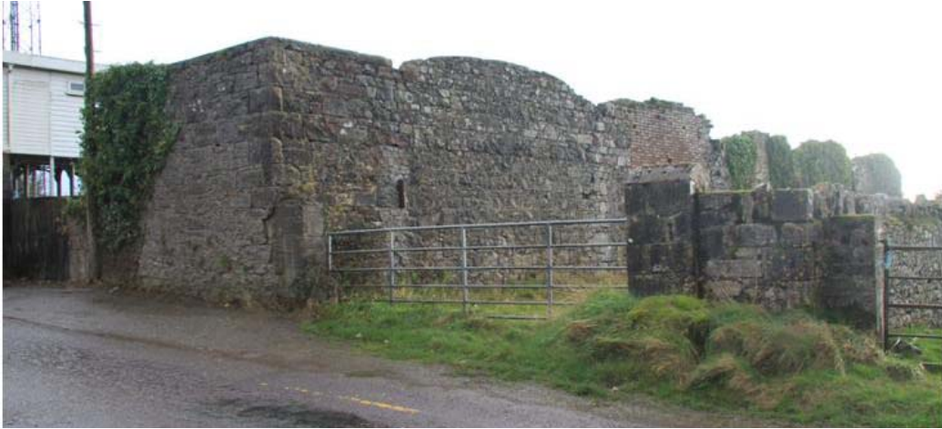
Plate 14: Western shed, seen from the road to the north-west
