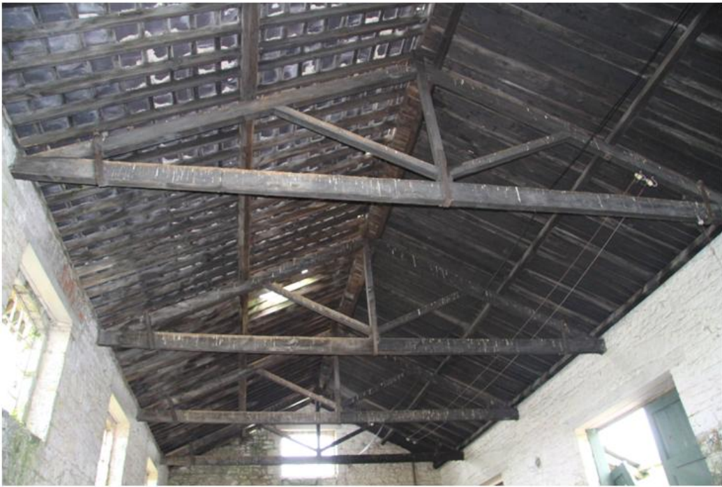
Plate 4: Internal roof structure of goods shed
