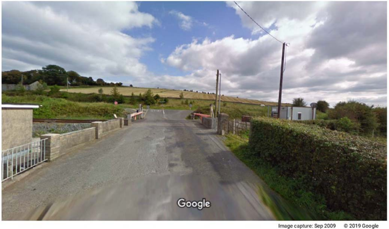
Figure 9.2 – Level Crossing XC215
