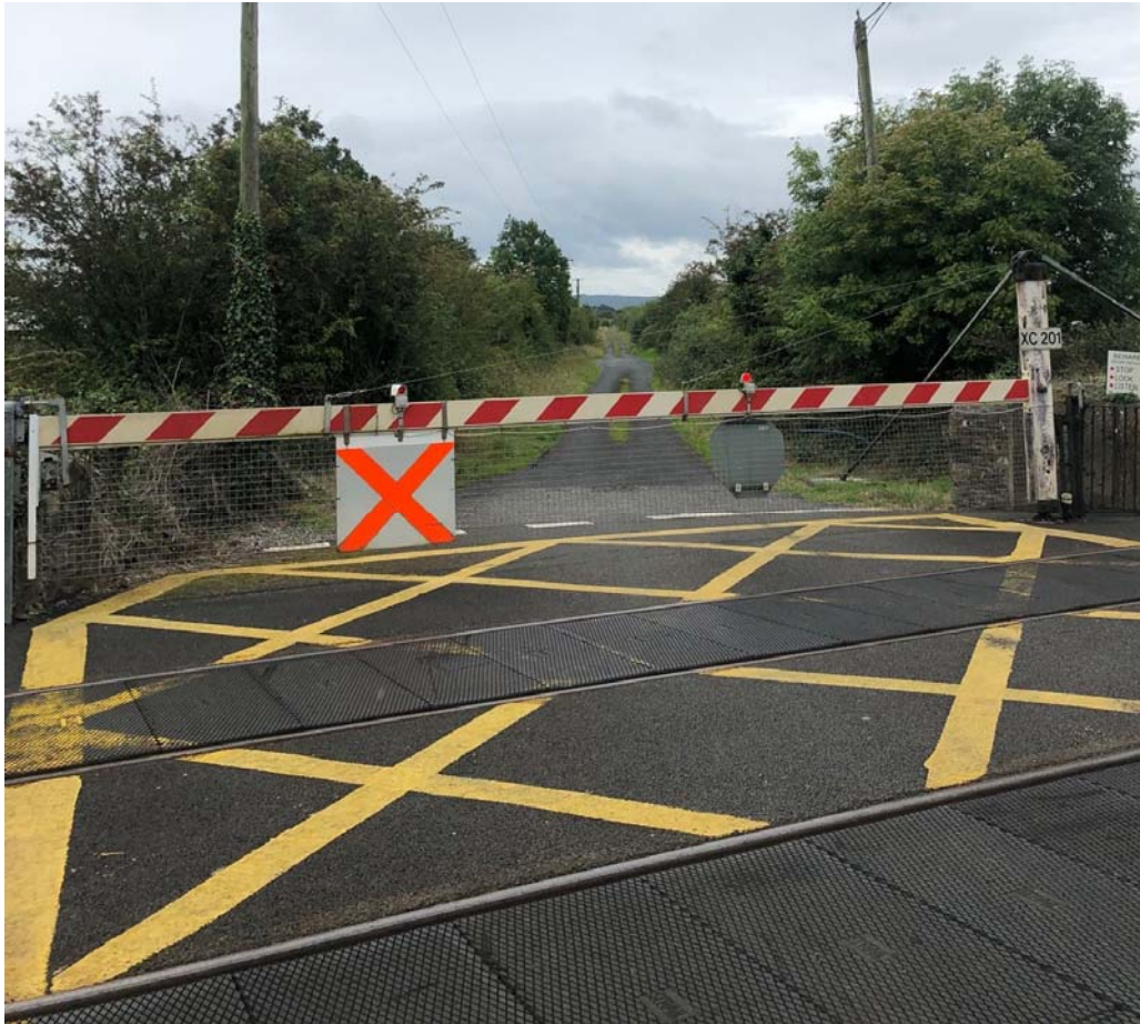
Figure 5.2 – Level Crossing XC201
