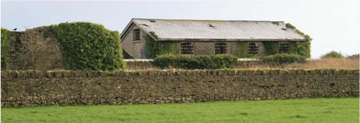
Plate 18: Western boundary wall
