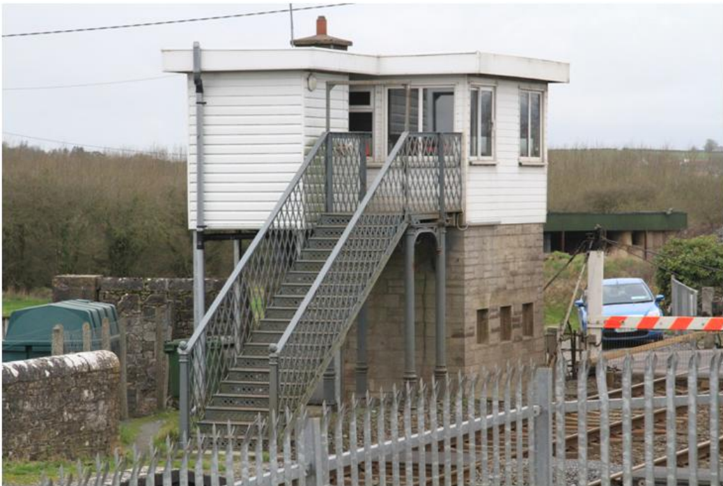
Plate 9: Signal box, with iron stairs
