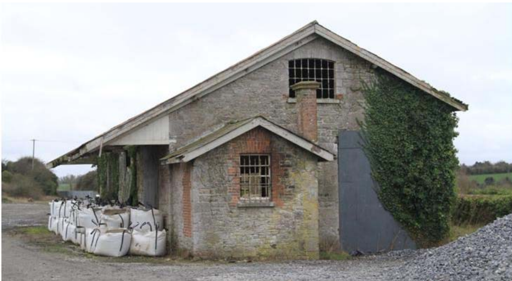
Plate 3: Northern gable of goods shed, with projecting office
