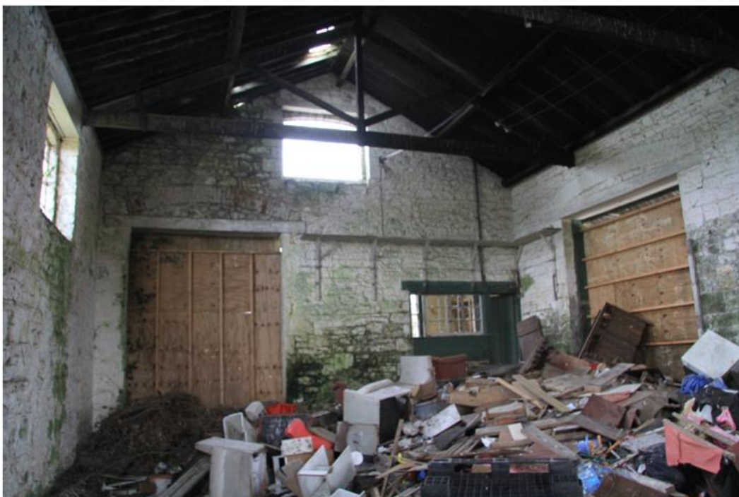
Plate 5: Interior of goods shed
