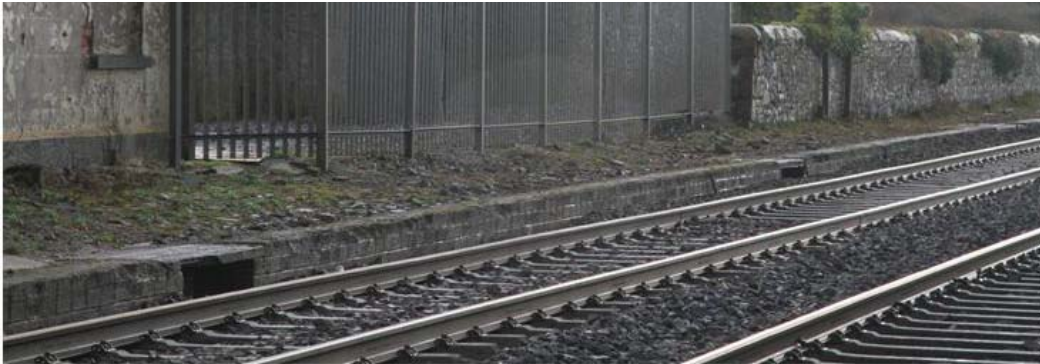
Plate 16: Down platform in northern part of station
