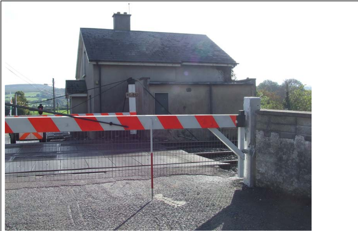
Plate 3 Station House facing east
