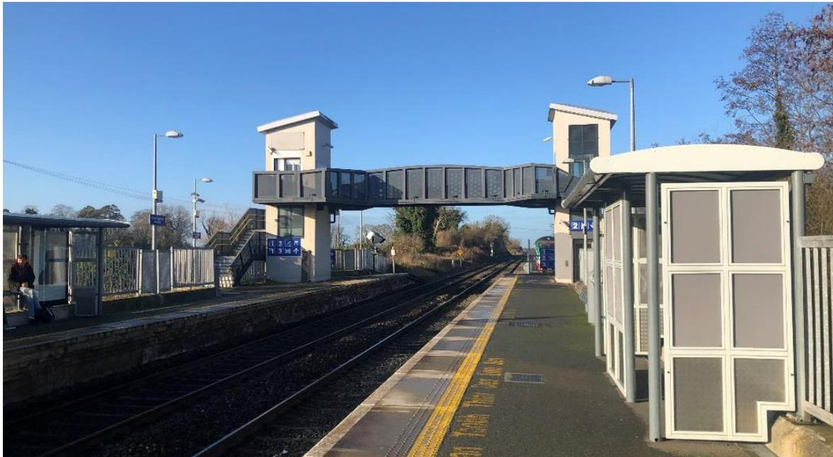
PHOTO 7 - Footbridge connecting both platforms with lifts.
