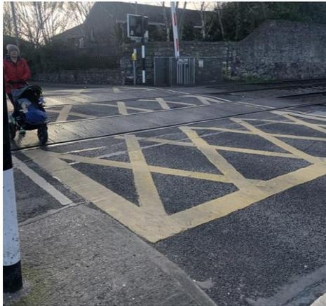
PHOTO 1 - Footpath markings for level crossing
