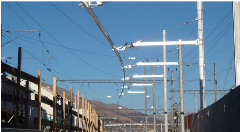
Figure 5-1 Typical Conductor Bar Installation
