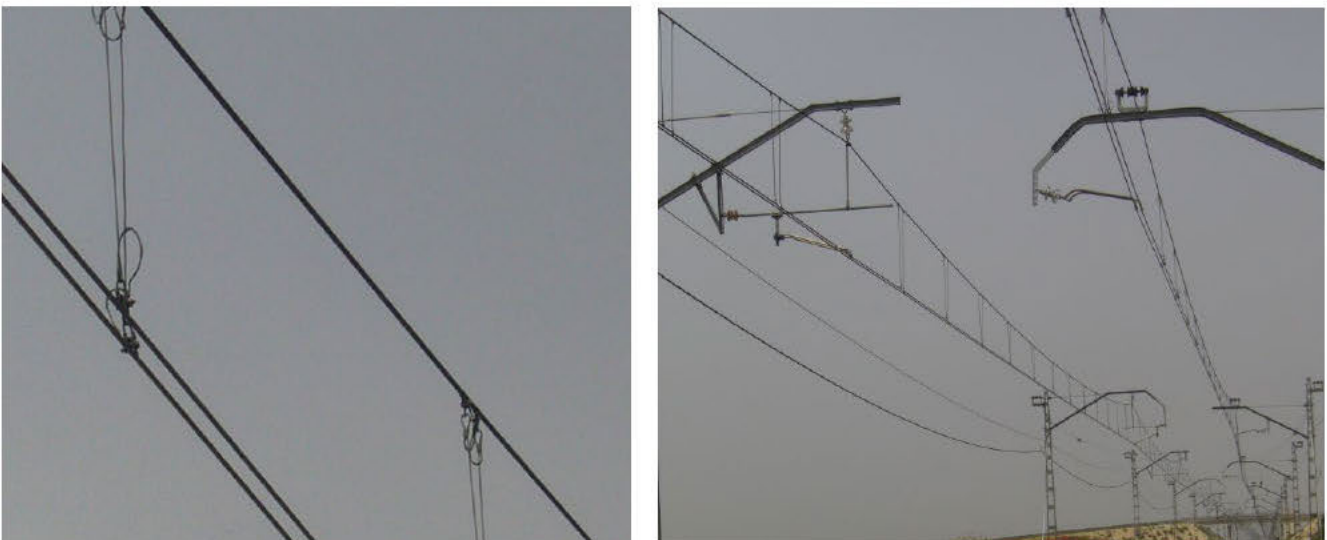
Figure 5-3 dual contact wire dropper arrangement(left) and registration support(right)
