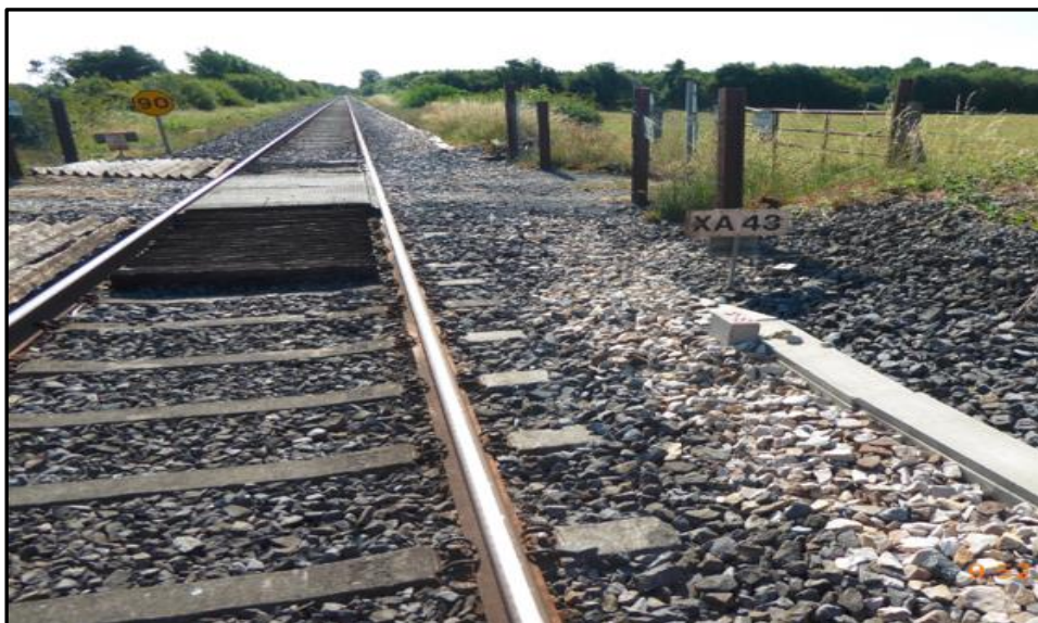
Figure 10: Post-incident image of LC XA043 showing missing Down side cess cattle grid. This view is looking towards Portarlinton. Note; the newly installed cable ducting.
