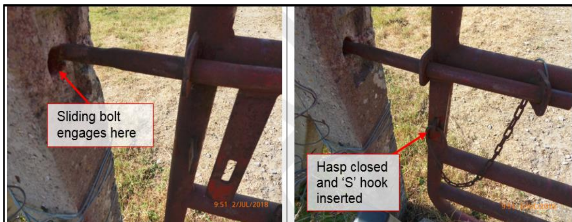
Figure 11: Post-incident images of the sliding bolt and hasp fastening arrangement of Down side gate at XA043.
