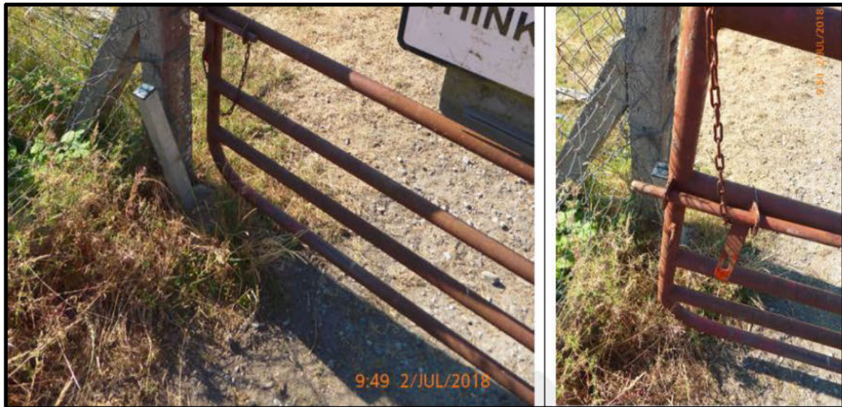
Figure 12: Post-incident images of the loose gate stop post on the Down side gate at XA043. This allowed the unfastened gate to open towards the railway.
