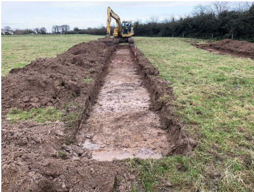
Plate 19: Test Trench 7, facing northeast
