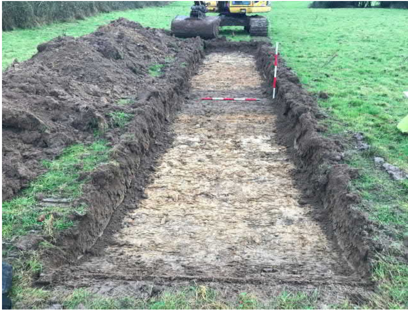
Plate 25: Test Trench 11, facing south
