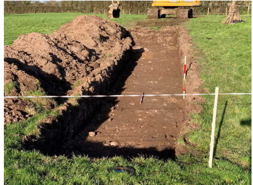
Plate 46: Test Trench 17, facing northeast
