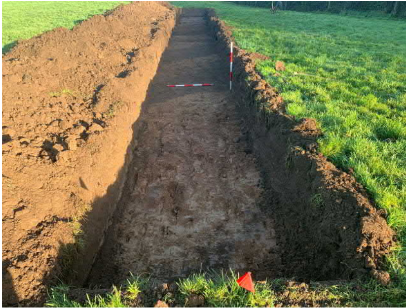
Plate 41: Test Trench 16, facing northeast
