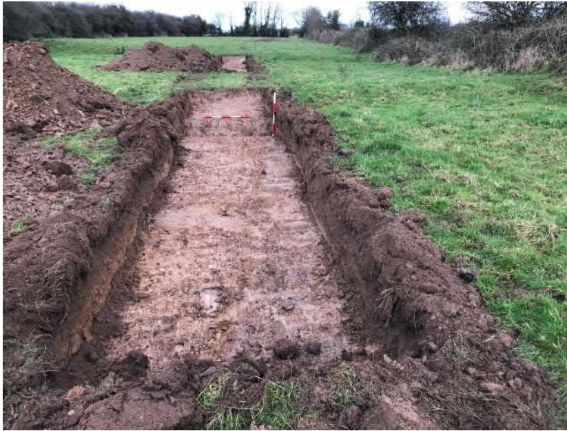
Plate 29: Test Trench 13, facing north
