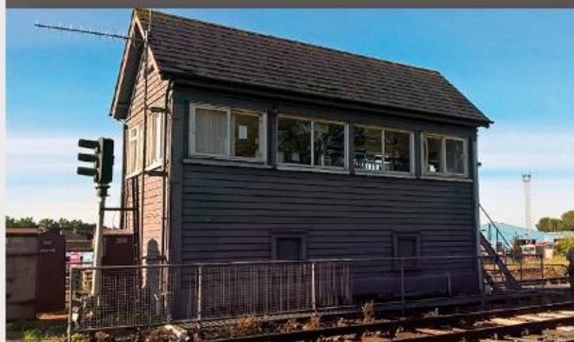
Old signal cabin at Limerick Check
