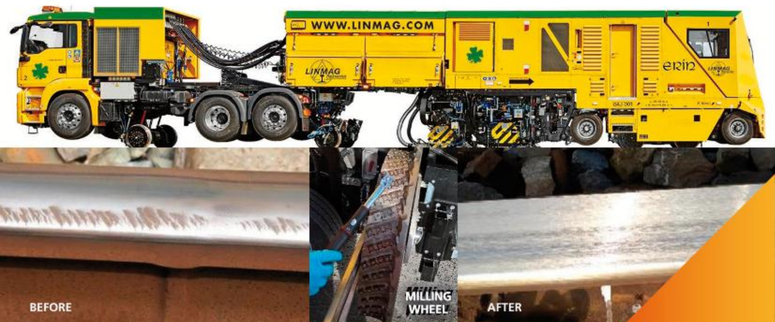
Removal of gauge corner cracking on the Cork line
