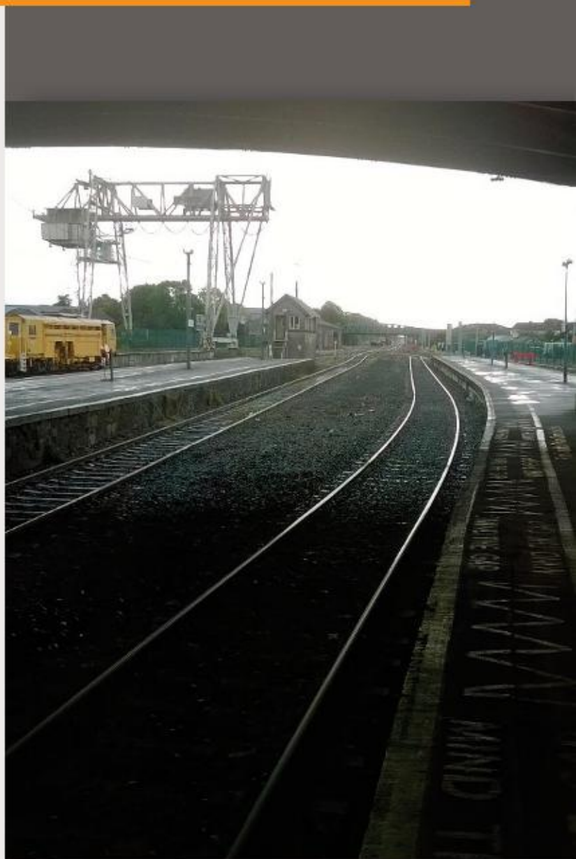
Reverse curve at platform 3 before reconstruction
