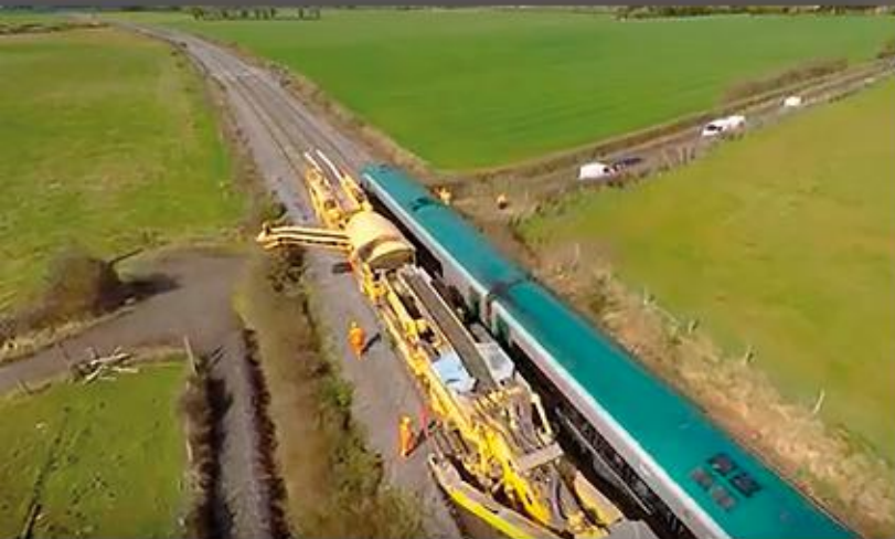
Figure 3 Ballast Cleaner working during SLW
