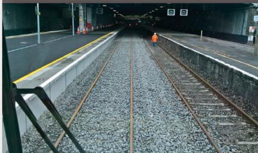
Approach to new platform 3 post reconstruction
