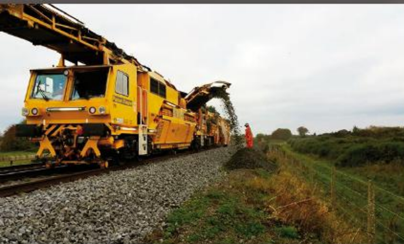
Figure 2 T781 Plasseur & Theurer Ballast Cleaning machine
