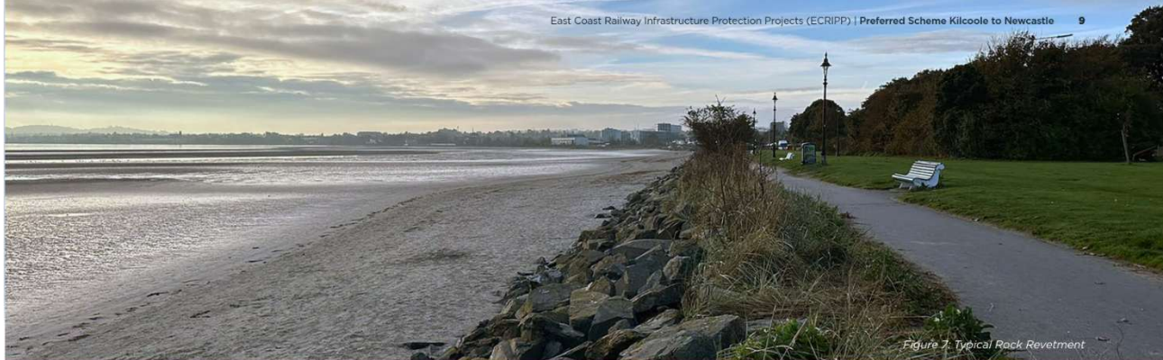
Figure 7: Typical Rock Revetment
