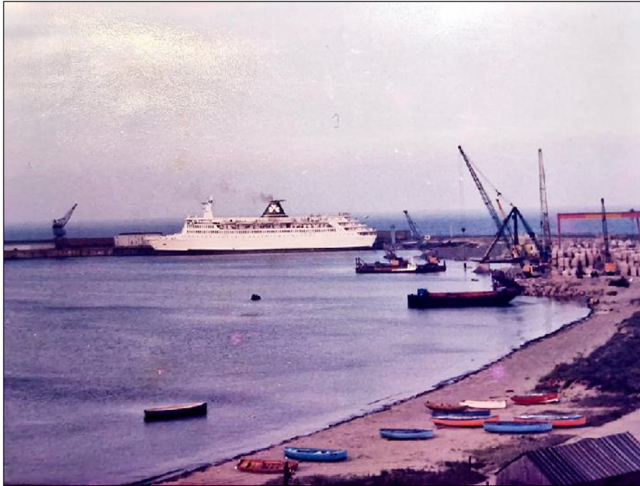
Plate 3: East-facing view of Rosslare Harbour, sometime in the 1980s, at start of reclamation of works along adjacent shoreline. Source: Rosslare Harbour, Old Photos, facebook page.
