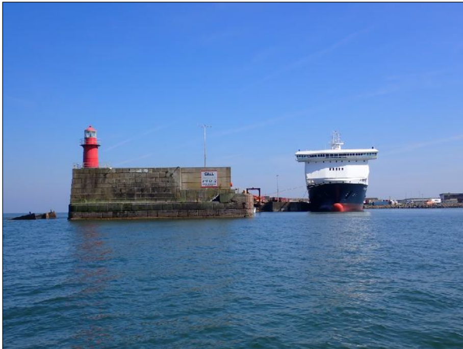
Plate 4: South-facing view of pier head with Ro-Ro ferry in dock at Rosslare Europort.
