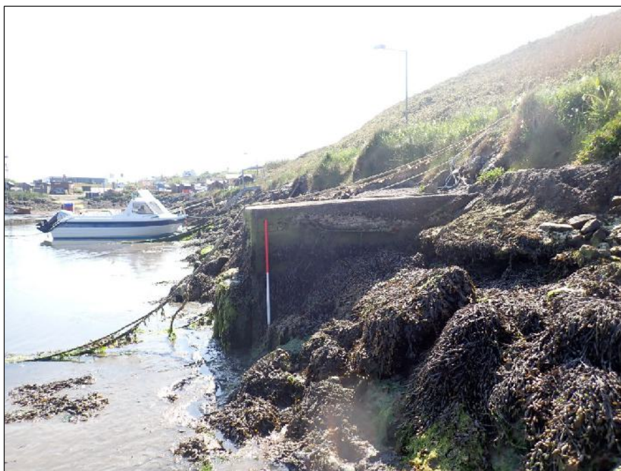
Plate 11: East-southeast view of rubble used to from southwest side of inner harbour area (1m scale).
