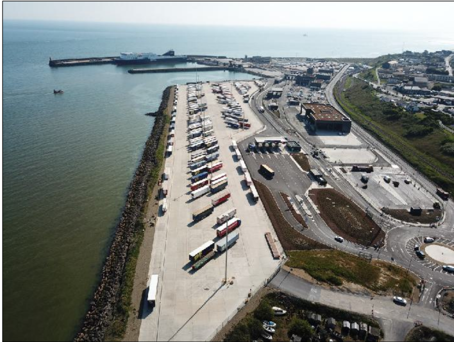
Plate 19: Aerial view of rock-armour revetment forming edge of reclaimed foreshore extending between the Small Boat Harbour and Rosslare Europort. Source: ADCO Drone.
