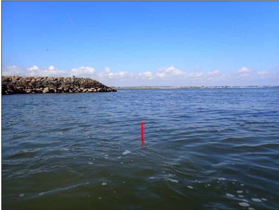
Plate 17: West-facing of entrance to harbour, scale delineating east side of sub-tidal channel (1m scale).
