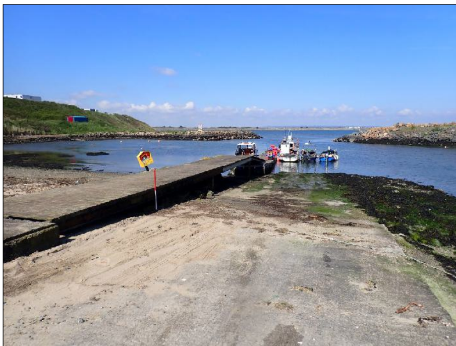
Plate 12: West-northwest view of concrete slip and pontoon structure (1m scale).
