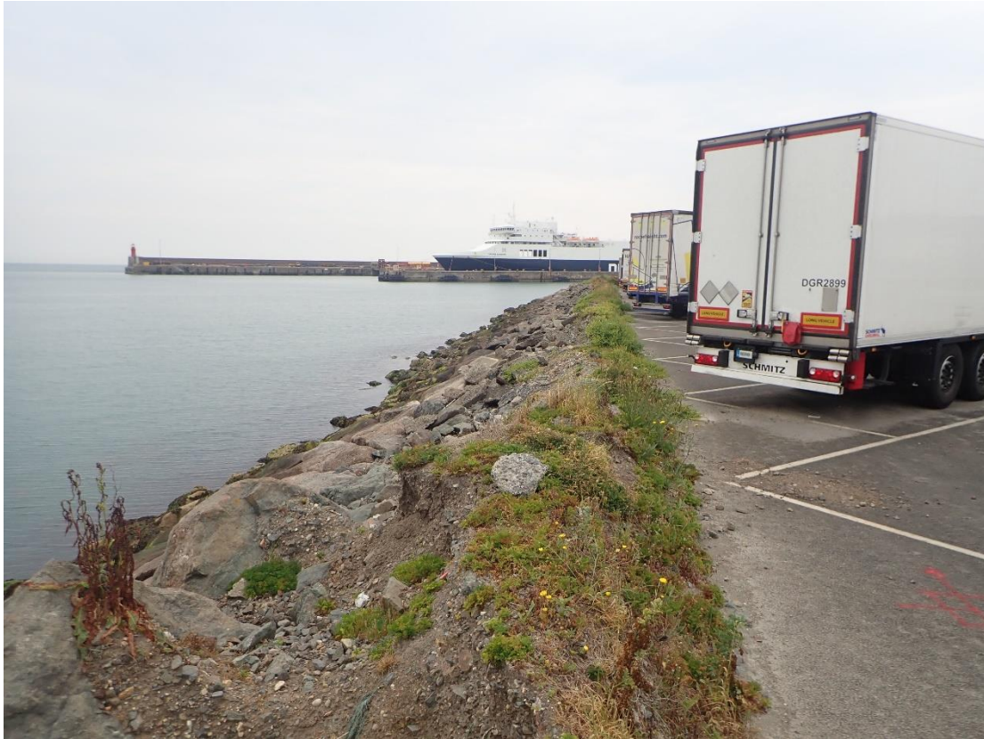
Plate 2: View looking east along shoreline from RoRo terminal towards pier head.
