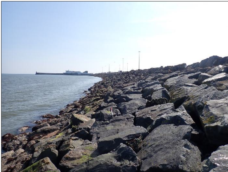
Plate 18: East-facing view along rock-armour revetment forming edge of reclaimed foreshore extending between the Small Boat Harbour and Rosslare Europort (1m scale).
