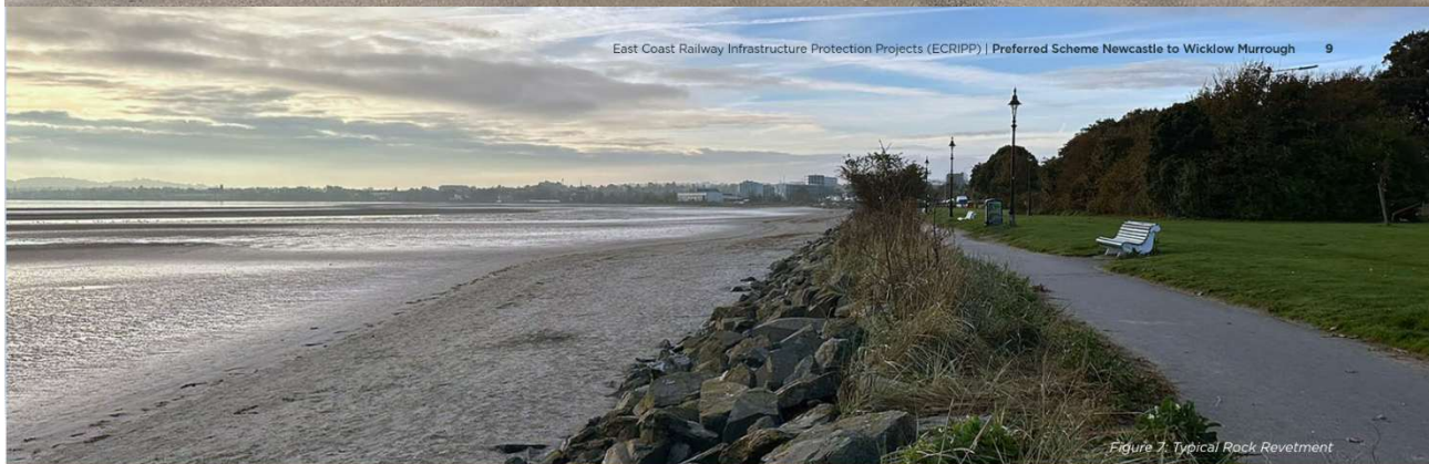
Figure 7: Typical Rock Revetment
