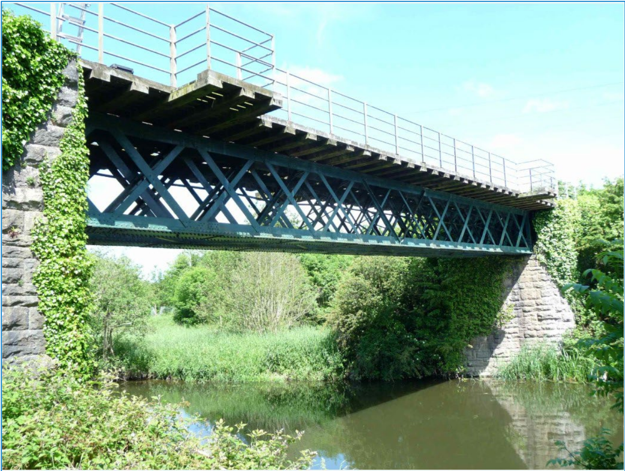
Figure 1-6: Blackwater River Underbridge
