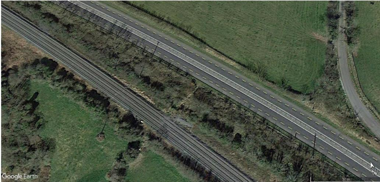
Figure 9-1 XC229 Buckley's Level Crossing
