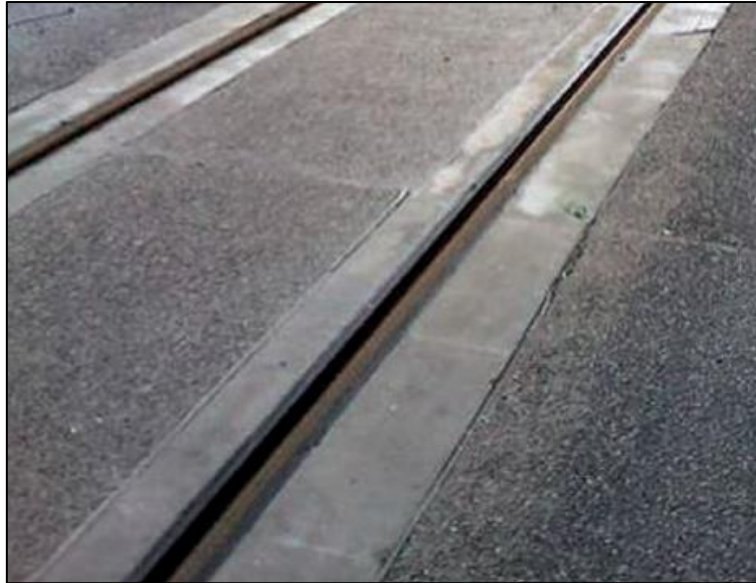
Figure 12-6 Embedded Rail in Slab
