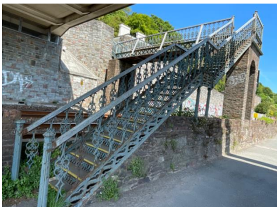
Figure 8-2 OBC409 pedestrian bridge on Lower Glanmire Road
