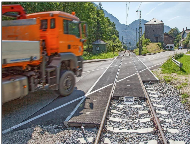
Figure 12-7 Strail Crossing Units at Road-Rail Interface
