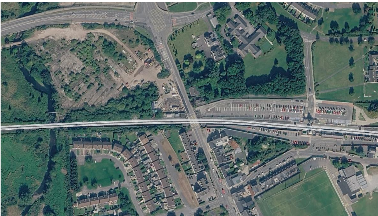
Figure 9-6 XY012 Mill Road Level Crossing
