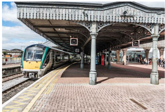
Figure 8-5 Kent Station Canopy
