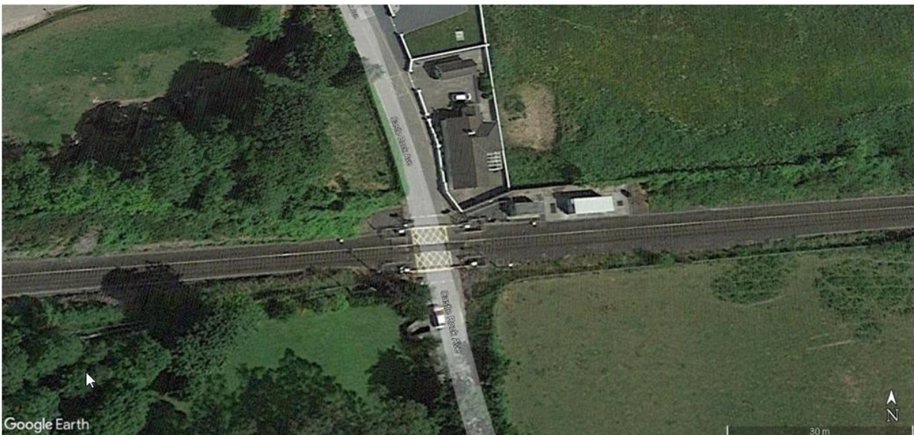
Figure 9-5 XY009 Water Rock Level Crossing
