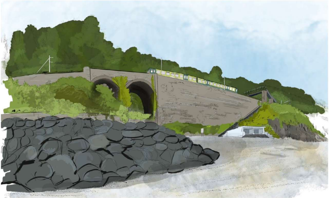
Figure 12: Illustrative view of rock revetments at Whiterock
