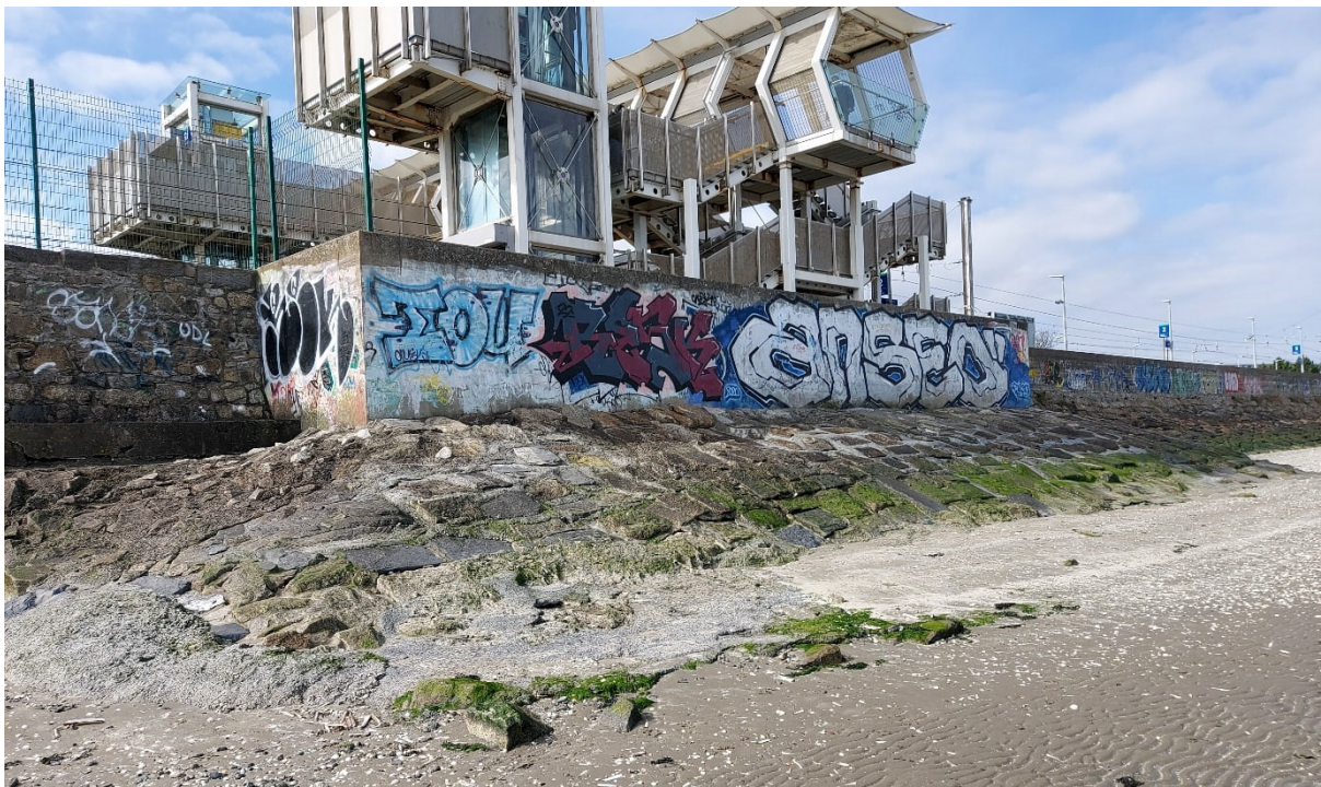
Figure 5 - CCA1-C: Booterstown station's coastal protection is very similar to the rest of the sub-cell, but with a higher upstand wall which protects the public from sea spray. The station is under additional pressure from storm events due to extending further onto the foreshore.
