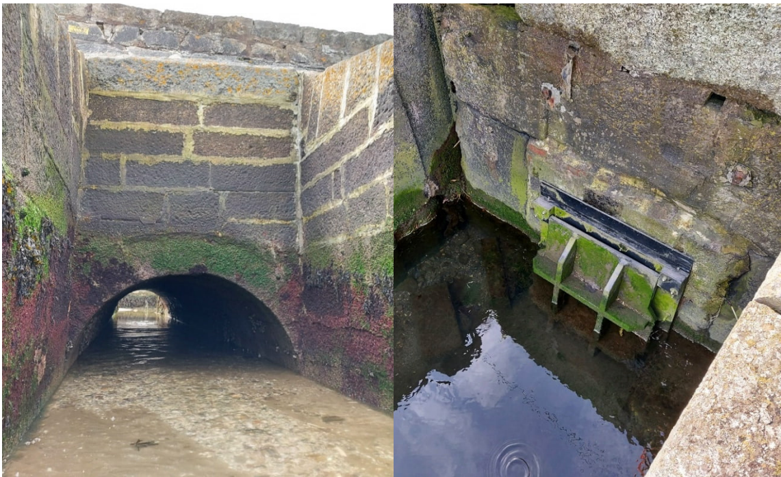
Figure 2 - CCA1-A: A stream located behind the railway and the existing surface water network which discharges to the sea through a series of culverts crossing the revetment. Some of these culverts include a flap gate to prevent upstream flooding during high tide.
