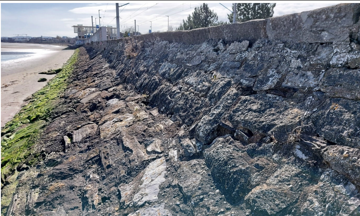
Figure 4 - CCA1-C: The sub-cell consists of a masonry revetment and an upstand wall. The area also includes Booterstown station, where an additional wall upstand has been added in recent years. The foreshore is sandy/silty and fully covered at high tide; algae are visible along the bottom of the defence.
