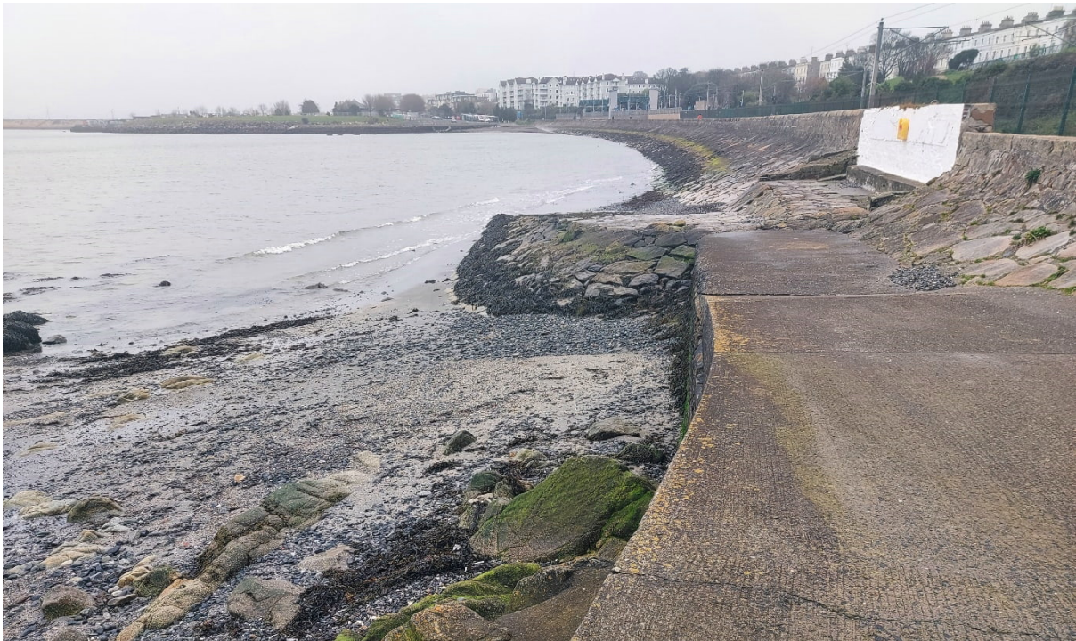
Figure 12 - CCA1-E: Throughout the sub-cell, the defence is a sloping masonry revetment with upstand wall. A walkway runs along parts of the sub-cell, with a short gravelly beach. There is no foreshore at high tide in the eastern half of this cell.
