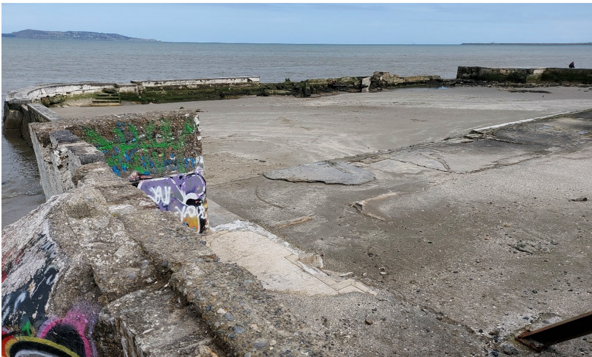
Figure 7 - CCA1-D: Historic baths are located within the northern part of the sub-cell, which are now disused. The remains of the baths are currently providing additional coastal protection, but a masonry revetment and upstand wall are located in front of the railway.
