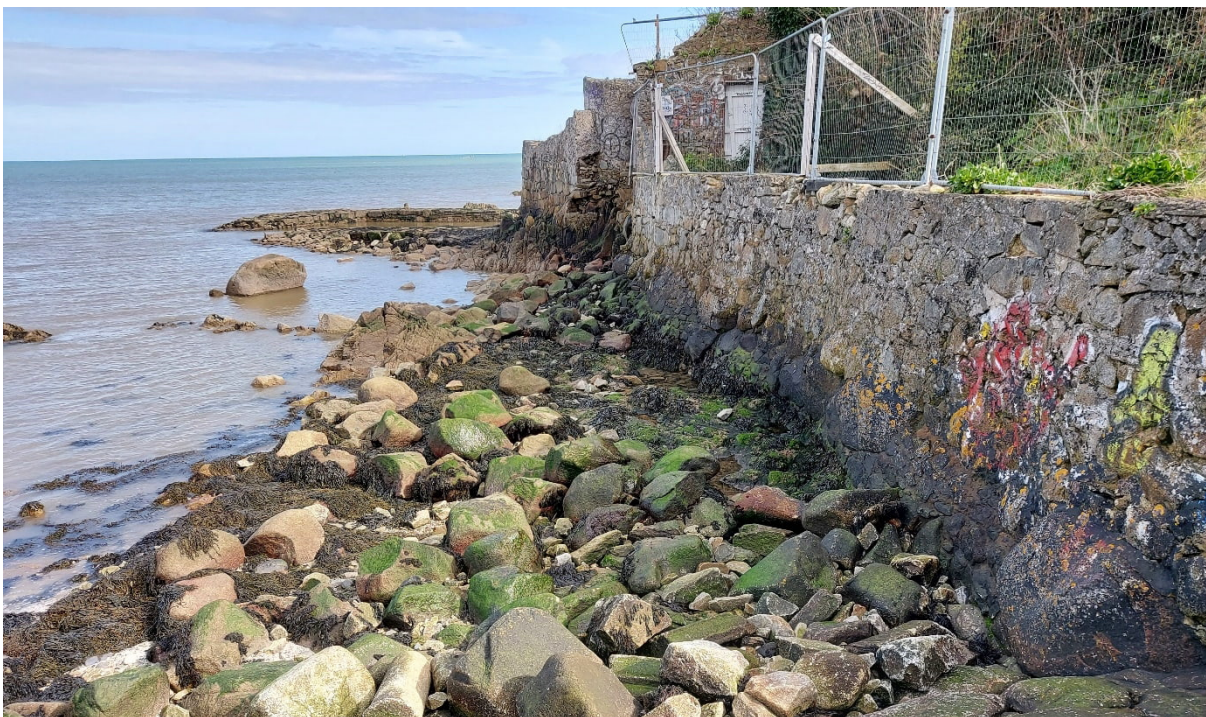
Figure 8 - CCA1-D: In the centre of the sub-cell, a small rocky headland with rocky foreshore is present and provides natural protection to the railway. A masonry wall is present along much of the headland.
