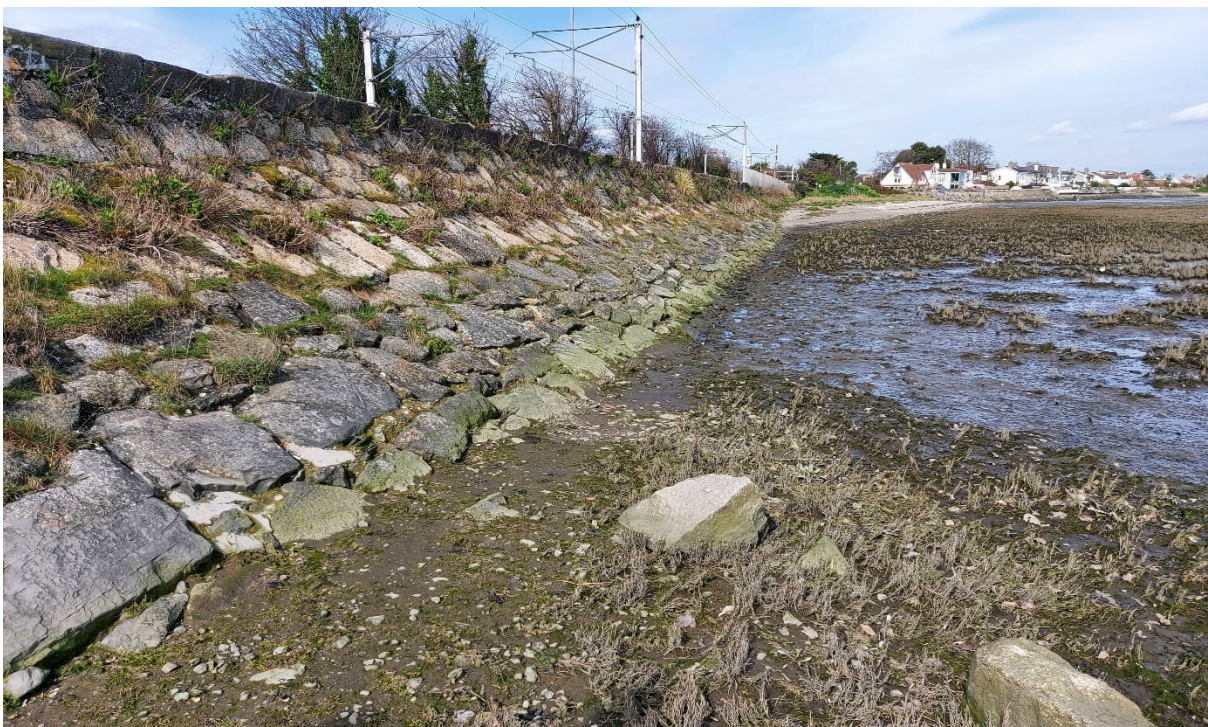
Figure 1 - CCA1-A: The sub-cell defence consists of a masonry revetment and an upstand wall. The northern half of the sub-cell is protected by a vegetated sand beach, while the southern half has muddy/marshy foreshore which is covered at high tide.
