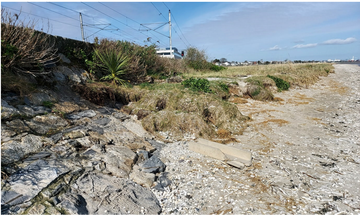
Figure 3 - CCA1-B: The sub-cell's engineered section is very similar to CCA1-A, with a masonry revetment and upstand wall close to the railway. In recent years, a sand spit has been accumulating in this area, providing additional coastal protection and habitat for birds.
