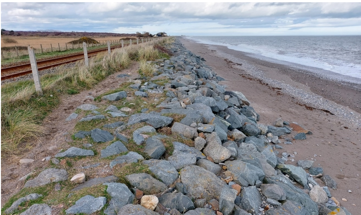
Figure 2 – CCA6.2-A: The second half of the sub-cell is protected by a 20m wide sand and shingle mix beach. At the back of the beach, there is some rock scour protection; the upper portion of the scour protection is vegetated. Evidence of localised erosion is visible.
