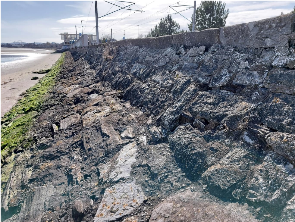
Figure 1-3. Typical defences from the Spit to Booterstown with the railway line directly behind the existing wall
