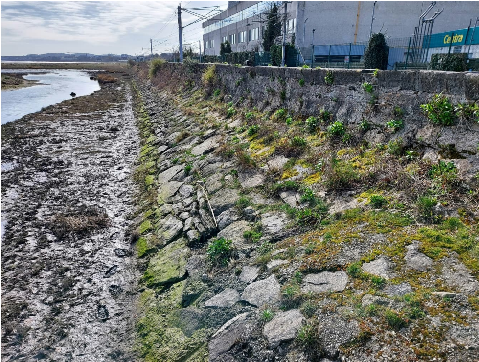
Figure 1-2. Example of defences at Merrion Gates showing the railway line directly behind the existing wall
