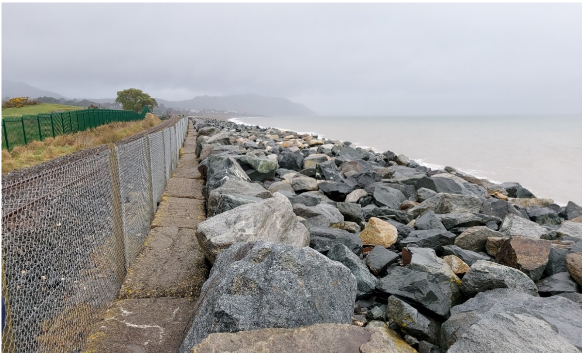
Figure 2 – CCA6.1-B: The sub-cell is a 2km steep rock revetment with concrete blocks at the back, located at the front of the local golf course. The railway here is located closer to the sea than in CCA6.1-A, resulting in more intense wave action. The rock is relatively large but has a broad variation in grading.
