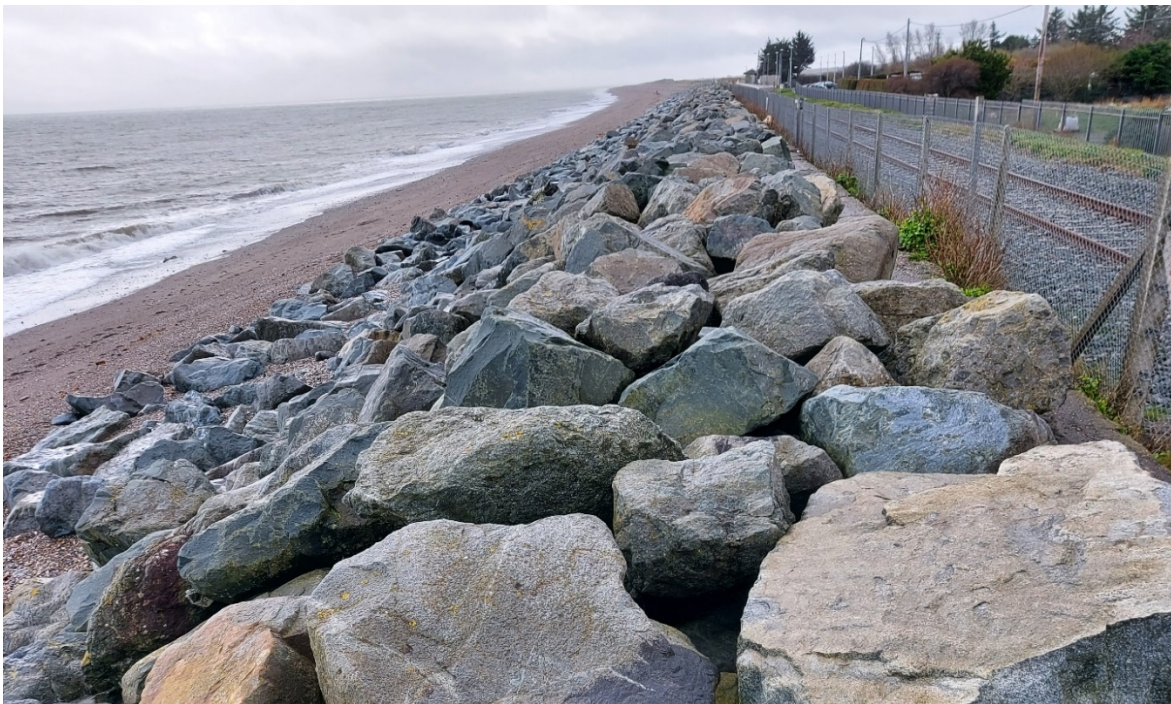
Figure 4 – CCA6.1-C: The sub-cell is a 1.8 km long section with rock revetment and concrete blocks at the back, located at the front of Kilcoole station. A relatively narrow and steep shingle beach is present in front of the revetment.
