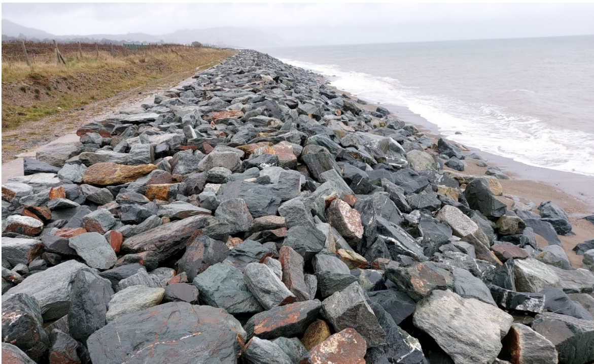
Figure 3 – CCA6.1-B: The rest of the sub-cell is also protected by a rock revetment and concrete blocks at the back. In this section, the rock used is of a smaller grading and is regularly displaced by wave action. The clearance between the sea and the track is large here, providing some additional protection to the railway.
