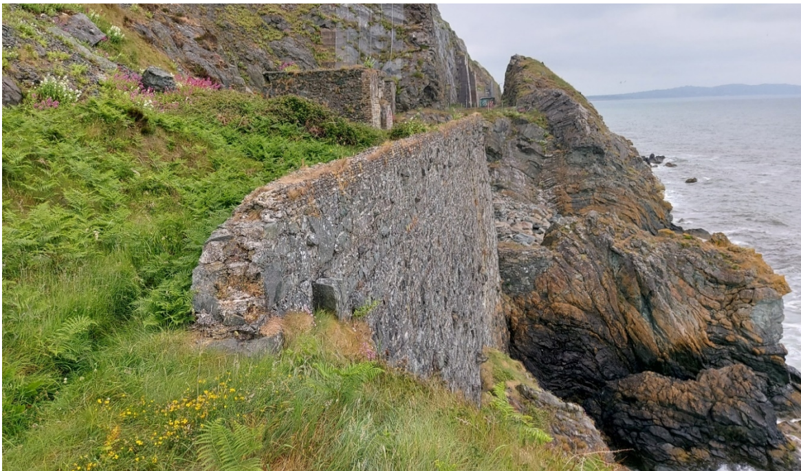
Figure 2 – CCA5-A: In some locations, masonry retaining walls have been installed to support the railway; these also serve as a coastal defence. In this image, the wall is located between two outcrops. In the upper section of the image, rock netting can also be seen, protecting the railway from debris and rockfalls.
