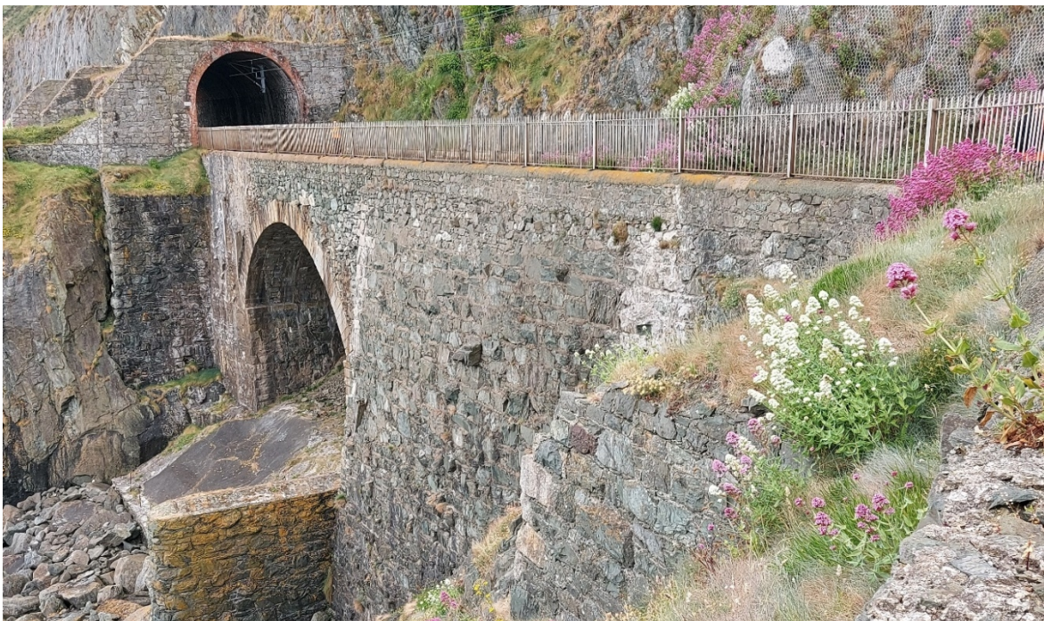
Figure 4 – CCA5-A: The railway within this sub-cell also goes through 4 tunnels, providing both coastal and rock fall protection. In this image, the entrance of Tunnel 1 is visible. A stone bridge/wall is located above the water level, and large boulders are located at the bottom of the asset.
