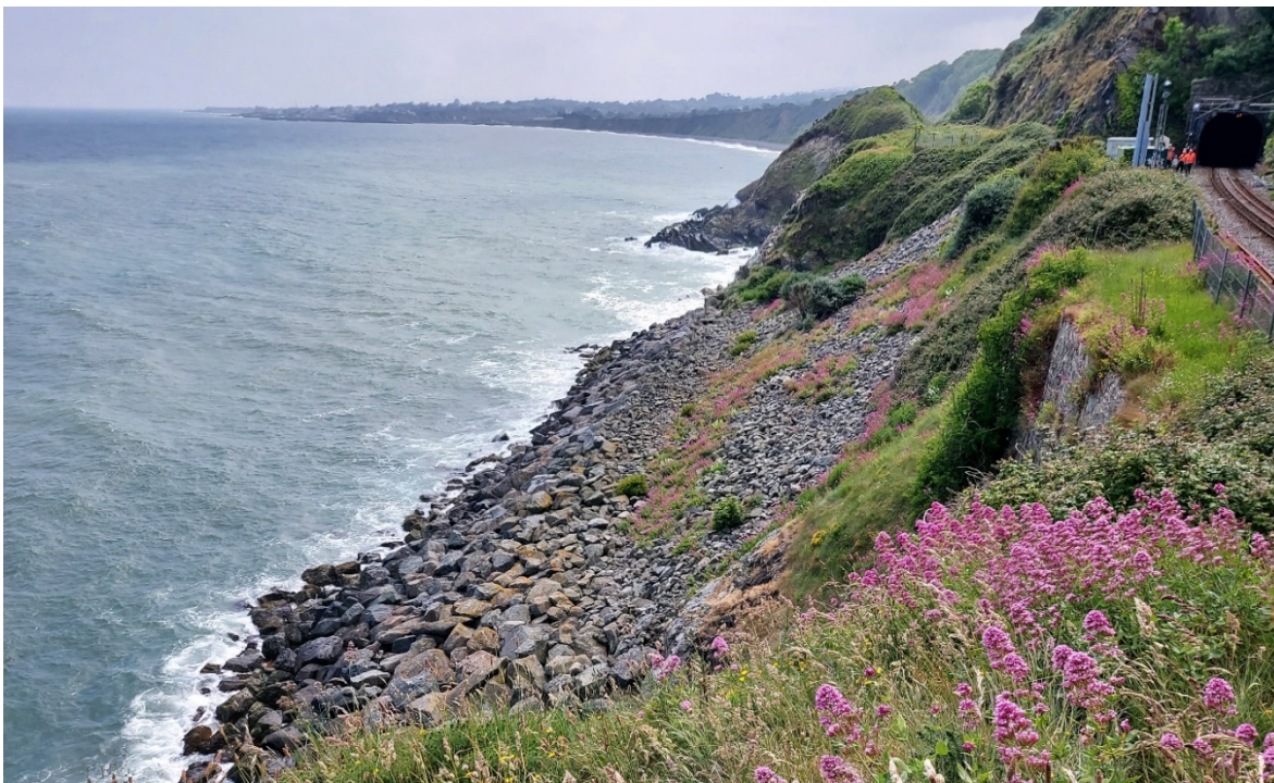
Figure 5 – CCA5-A: The entrance to Tunnel 4 can be seen here, with a rock armour protecting the toe of the asset. The boulders are very large and provide efficient coastal protection. Vegetated slopes are present between the rock armour and the railway. A retaining wall is also present on the right-hand side.
