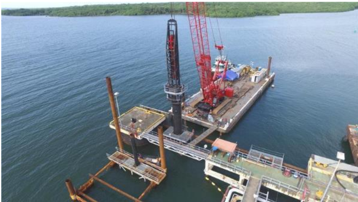
Figure 6.12: Example of impact piling in marine conditions 3
