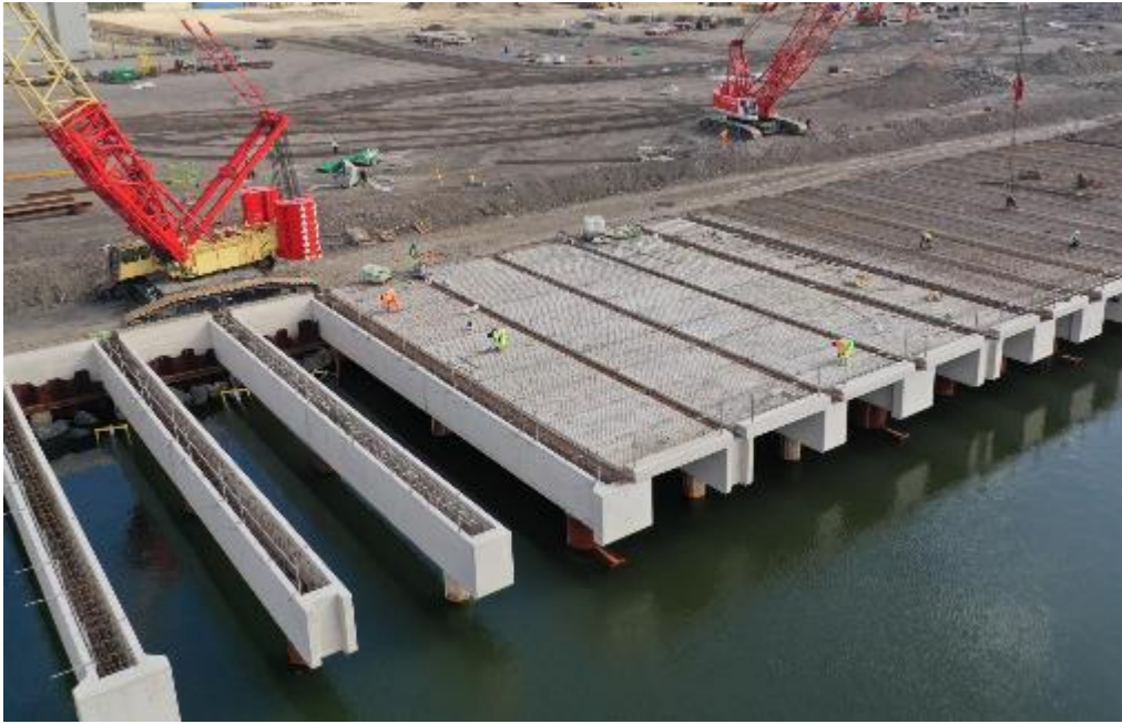
Figure 6.11: Example of open piled quay construction at Port of Dundee 2
